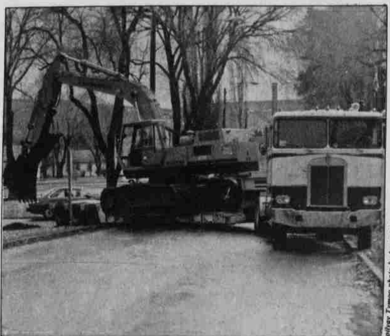
A simple 90-degree turn resulted in an hour-and-a-half traffic jam at the corner of Paiute and Wasco November 24. A Downing Construction Company truck, driven by Keith Gibson, failed to negotiate the turn, the trailer high centered and was unable to back up or pull forward. The trailer had to be unloaded before the trailer broke free. It added some excitement to an otherwise dull Monday morning.
