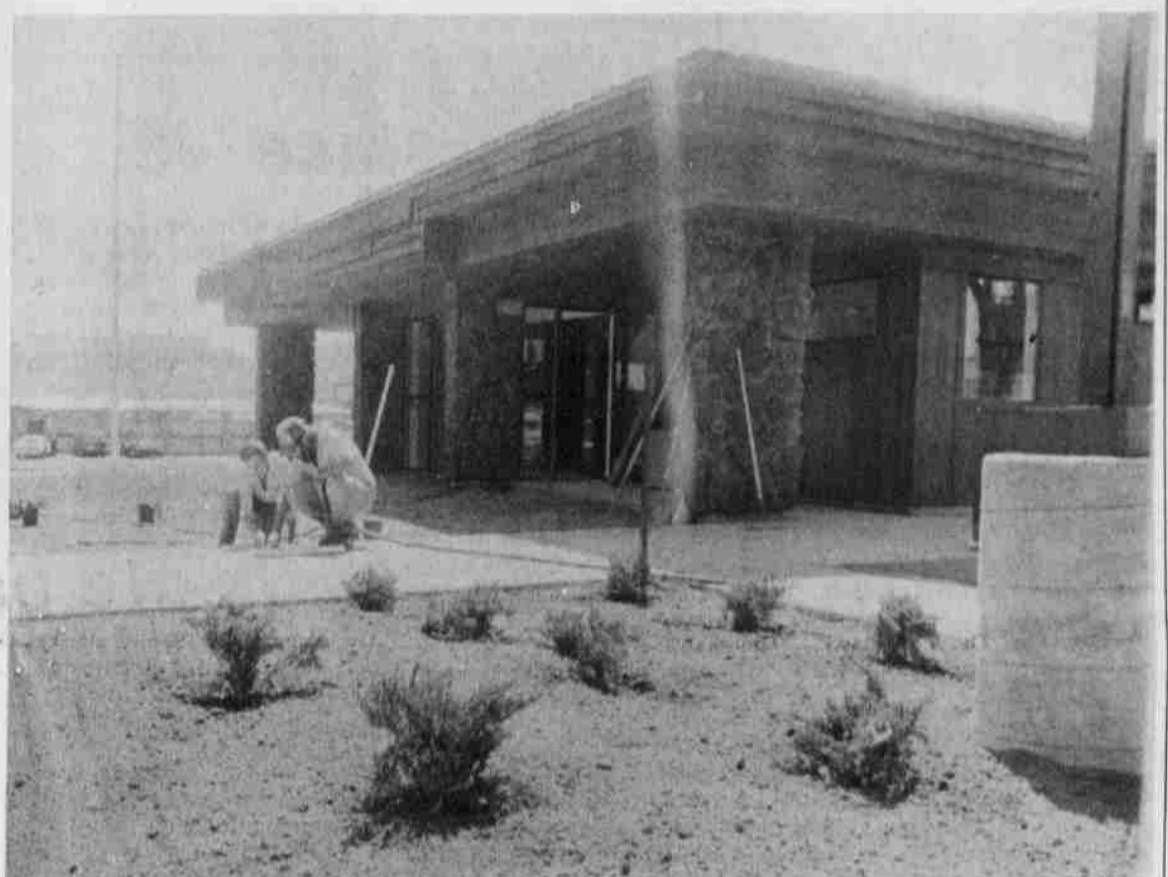
Checking the bluepring plans for yard
