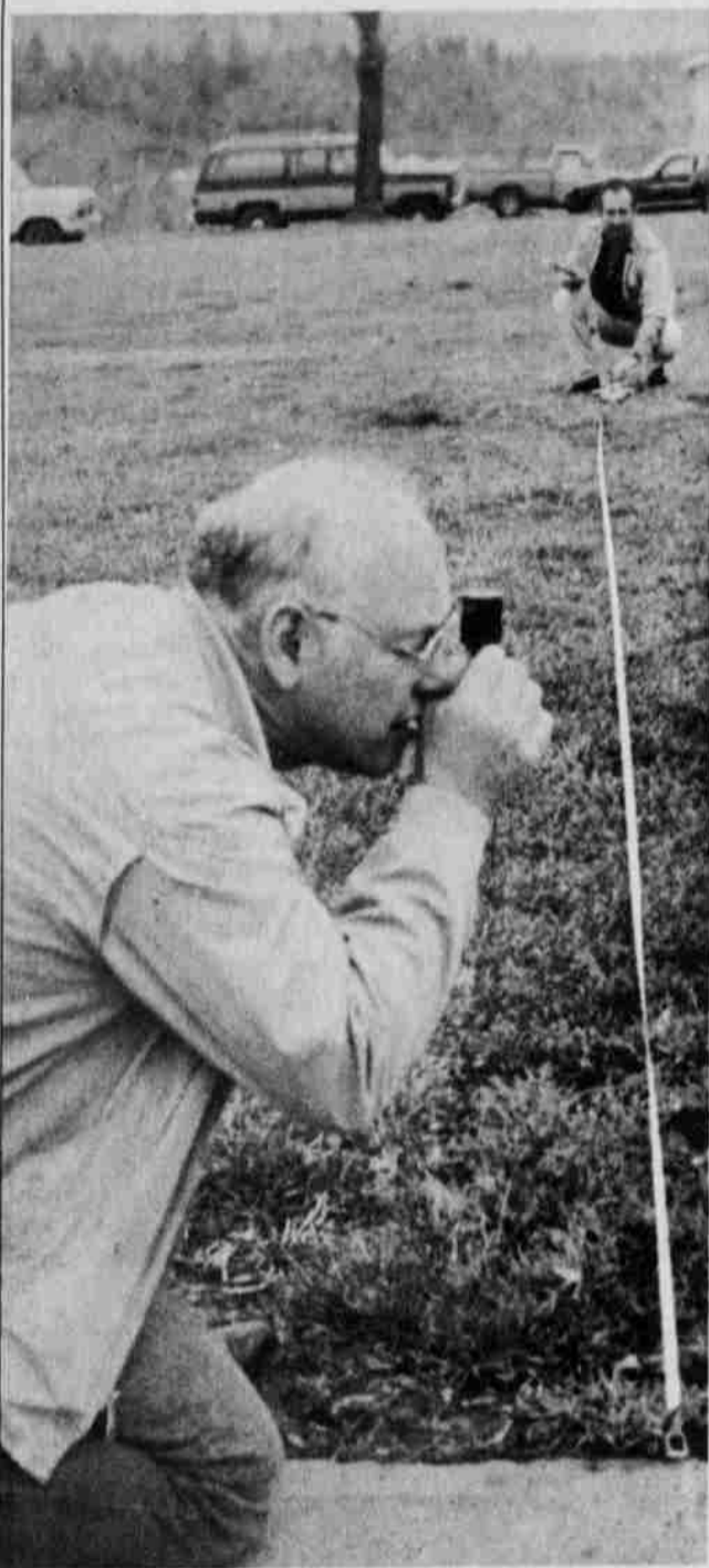
The onset of the project—surveying.
