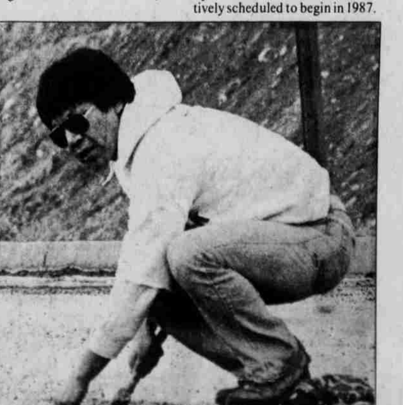
Holding driving nail used as point marker engineering technician Leo Hellon helps in preliminary road work.
