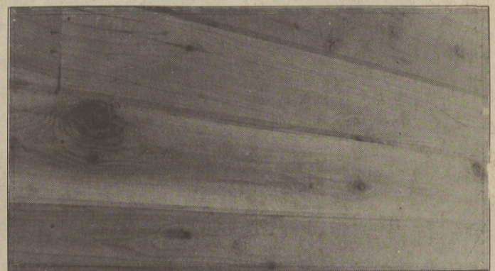
Cedar paneling adorns walls and ceilings of both old and new Longhouse structures.
