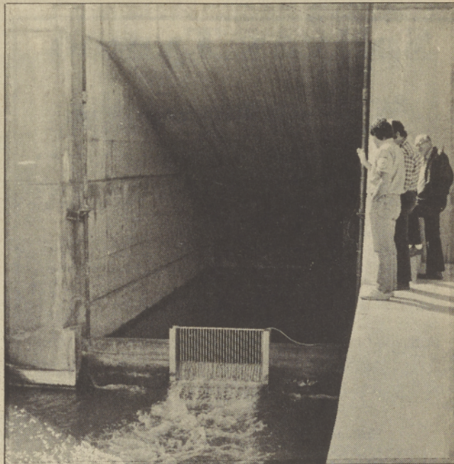
COUNTERS INSTALLED—Counting devices recently installed in fishways at Pelton Reregulating dam will help determine which entrance fish are utilizing. If fish runs are not affected, water will be used to generate power.
