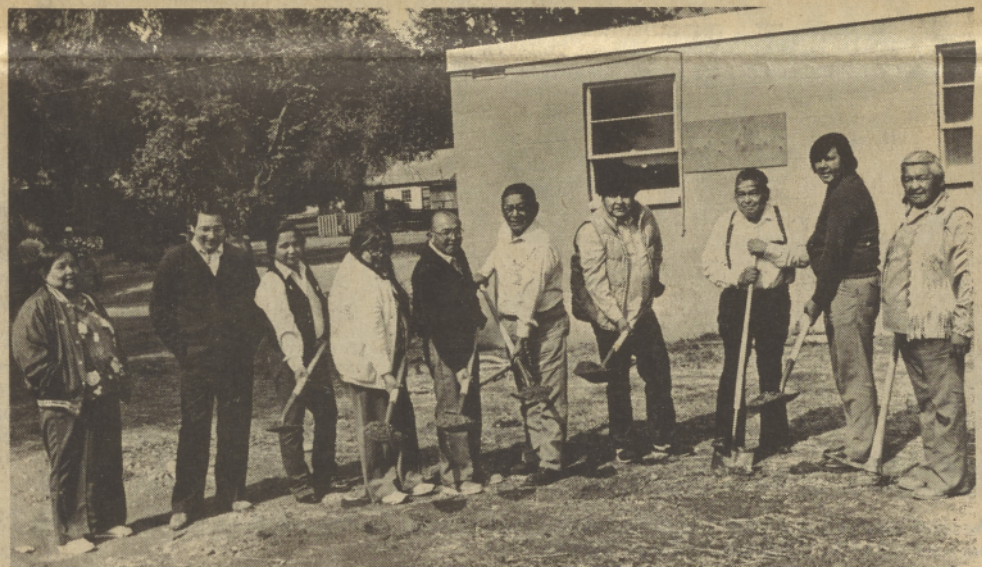
Construction began on improvements for the existing tribal jail. Tribal members rejected the idea of building a new facility in a referendum. The improvement is being funded by the Bureau of Indian Affairs who now holds title to the building. The project will be completed in the fall of 1985.
