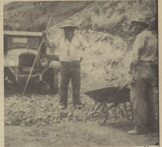
Machinery used to work on the road from Warm Springs to Mecca during this era. . manpower, a wheelbarrow and a rake.
