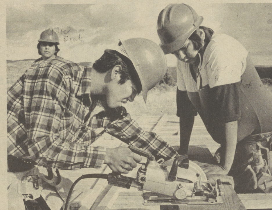
Cuts are made after measuring for fit. Mistakes do happen but with concern for accuracy they don't occur too often Hamley Danzuka (left) and Waldon Winishut (right) use circular saw.
