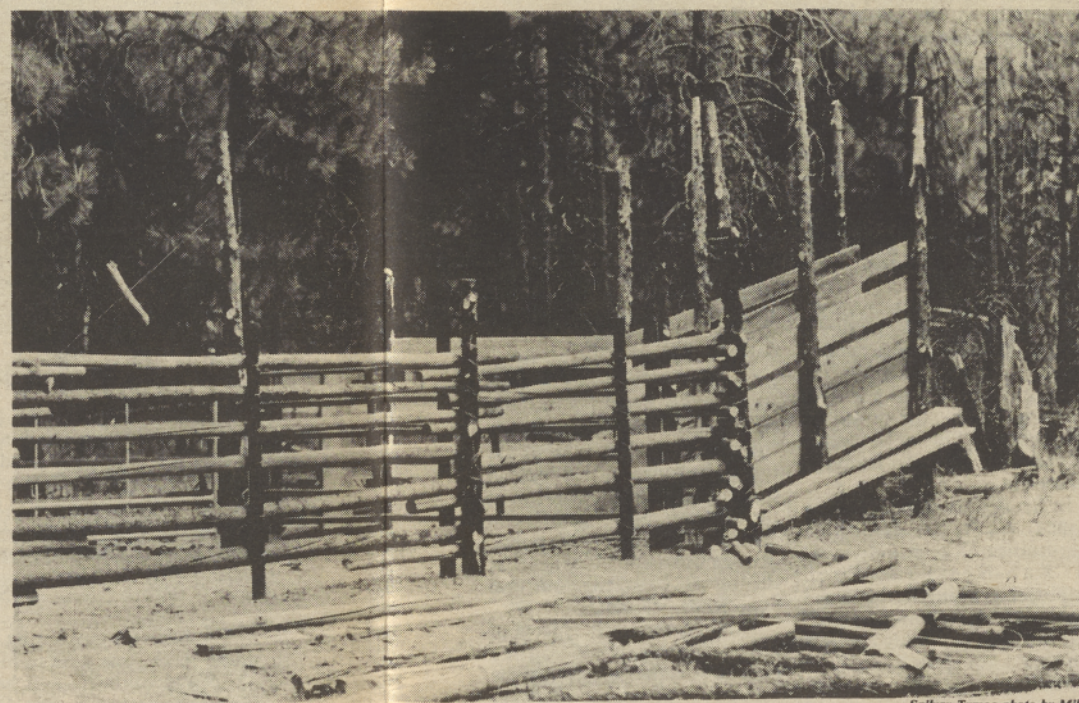
A finished product, the Seekseequa Corral, was one of 12 corrals that were rebuilt or repaired by Jobs Bill monies and crews. Spikey Tymoo photo by Miller
