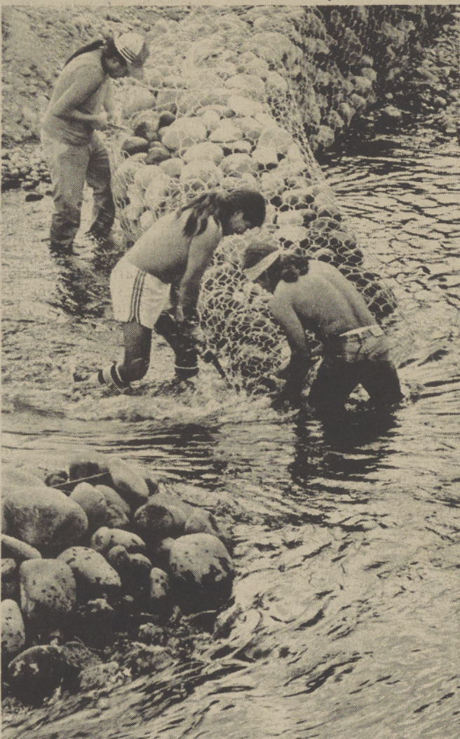
Tilden McDonald (left), Casey Jackson (center) and Austin Smith (right) deposit stones in wire mesh baskets while building gabions to channel water in Shitike Creek.
