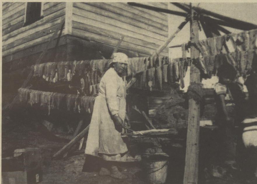
Watsuts, on the Columbia River near The Dalles, was Annie's birthplace. She returned there many times with her family to catch and prepare salmon. Some of the buildings at Watsuts are currently located near The Portage Inn in The Dalles.
