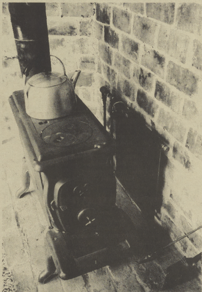
When the day is cool and overcast coils located next to a wood burning stove can provide heat needed to warm a home's water
