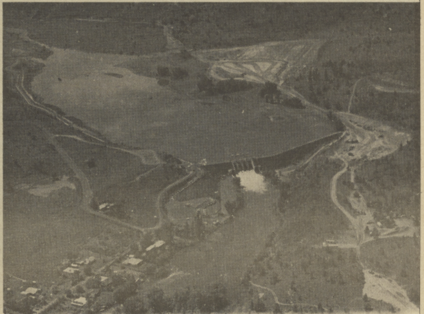
Tribal Power —Work began on the hydroelectric project in the spring of 1980. The powerhouse is the first federally licensed power project owned by an Indian tribe.
