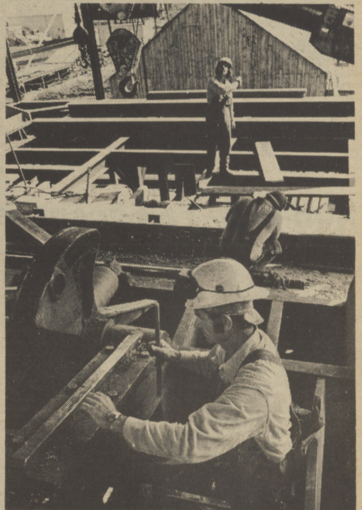
W.S.F.P.I. managers Ralph DeMoisy and Bob Macy oversee construction at the sawmill, the site of massive renovations. While the log-turner is removed (below) the sawmill walls are extended to accommodate the new carriage and headrig assembly, (left). Spilyay Tymoo Photos by Stowell
