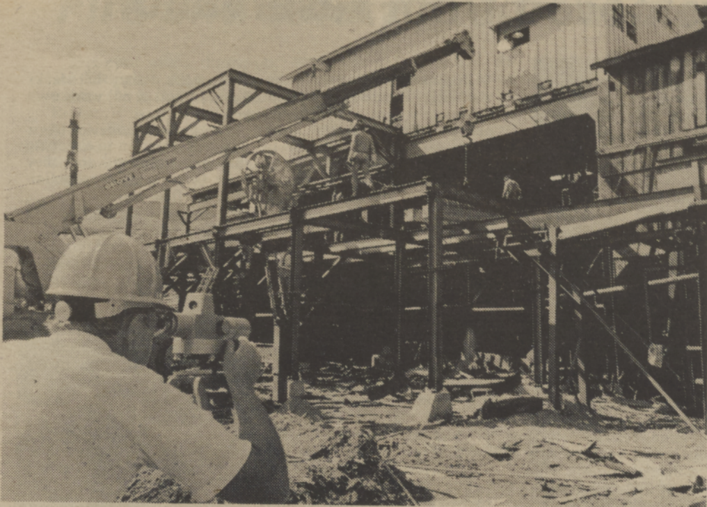
W.S.F.P.I. managers Ralph DeMoisy and Bob Macy oversee construction at the sawmill, the site of massive renovations. While the log-turner is removed (below) the sawmill walls are extended to accommodate the new carriage and headrig assembly, (left). Spilyay Tymoo Photos by Stowell
