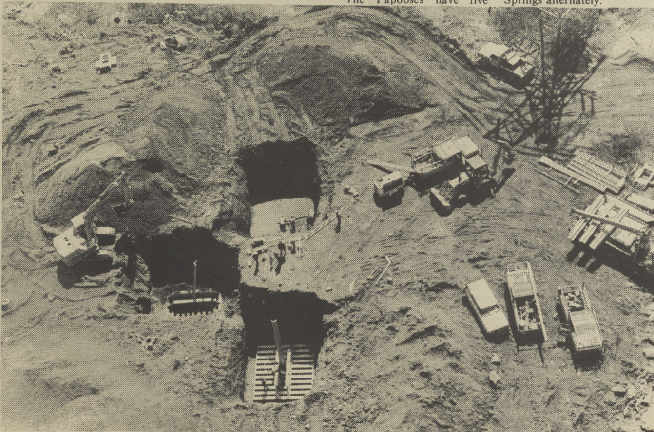
FOOTINGS AND FOUNDATIONS - Since mid-April, Bonneville Power Administration crews have been digging the foundations and placing footings for the 125-foot transmission line towers which will cross 16 miles of the northwest corner of the reservation. The work is now approaching Highway 26 near HeHe Butte. The 500-kv double circuit transmission line and towers should be up by October 1980 when the project is scheduled for completion. Spilyay Tymoo Photo by Rangila
