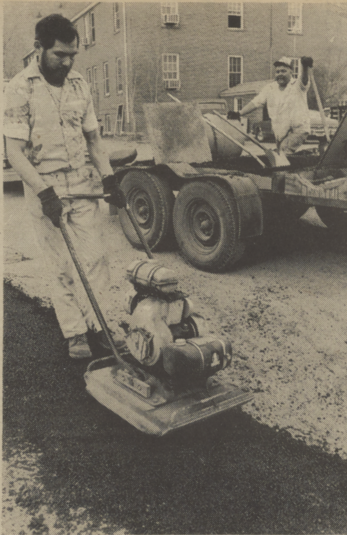
PATCH JOB - Roads on the reservation have suffered from the wet, freezing weather. For the last few weeks Terry Courtney, Jr. and Bobo Miller of the B.I.A. Roads Department have been patching potholes around the community and on the highways. This is the most patching they can remember doing. Spilyay Tymoo photo by CDS
