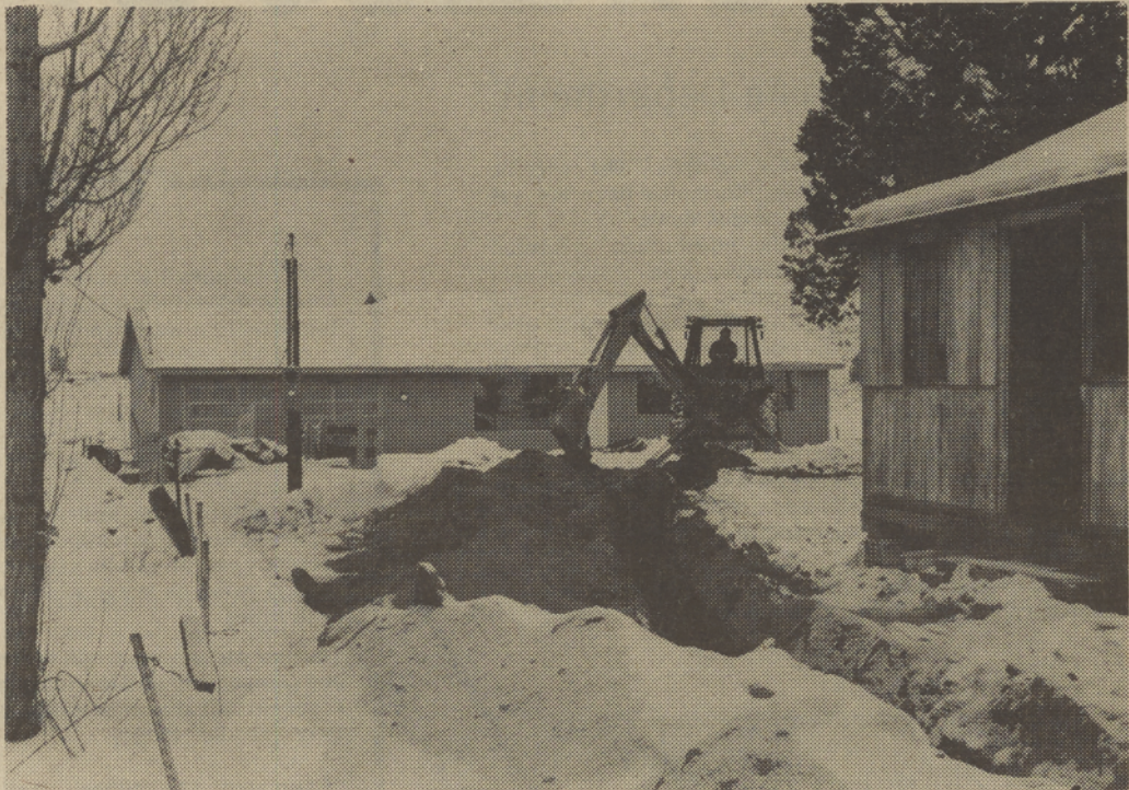
ALMOST READY — The new Adair home soon to be occupied by Carol and Fred Muniz, located in Seekseequa, was recently supplied with the ditch that will carry the water supply from their well 100 yards away. Luckily, the exterior work on the home was finished before the weather turned cold, as it often prohibits construction. The Muniz' began the paper work on their home in late August and hope to be moved in within a month.
