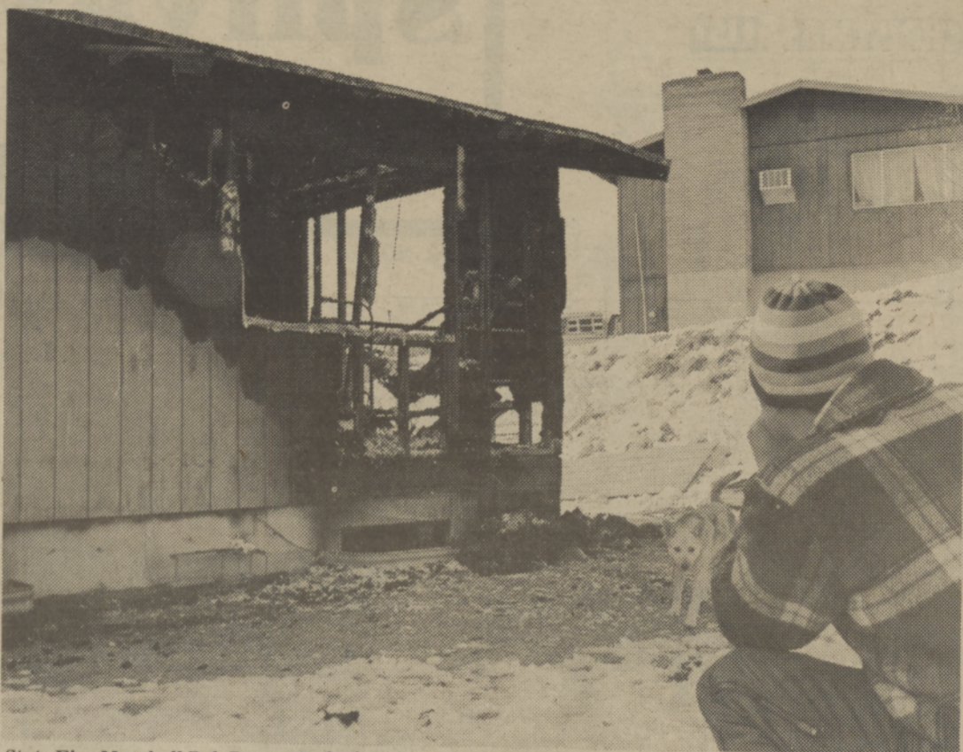
State Fire Marshal Bob Berney took pictures of Hazel Suppah's house which burned early November 26. Fire started in the rear basement bedroom and spread up the stairwell in the West Hills Split-level.
