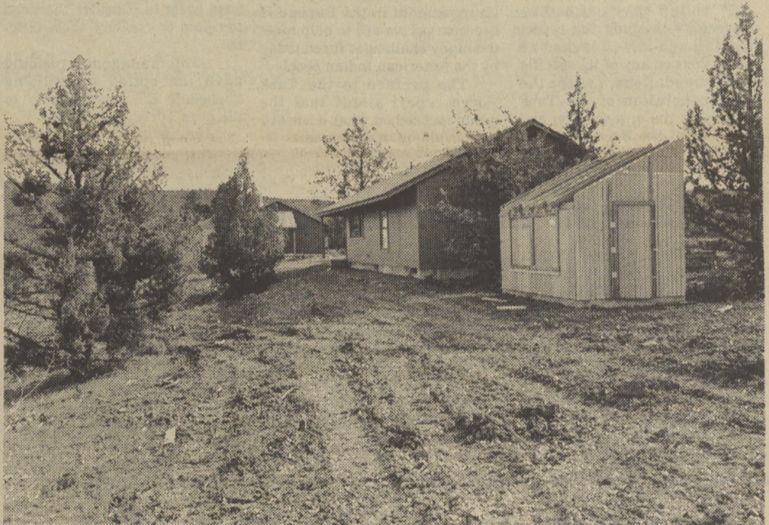
Each of the senior citizen houses has an individual smoke-house (right) as well as a carport. A HUD project, the homes should be ready for occupancy sometime this summer. Sandy Rangila Photo
