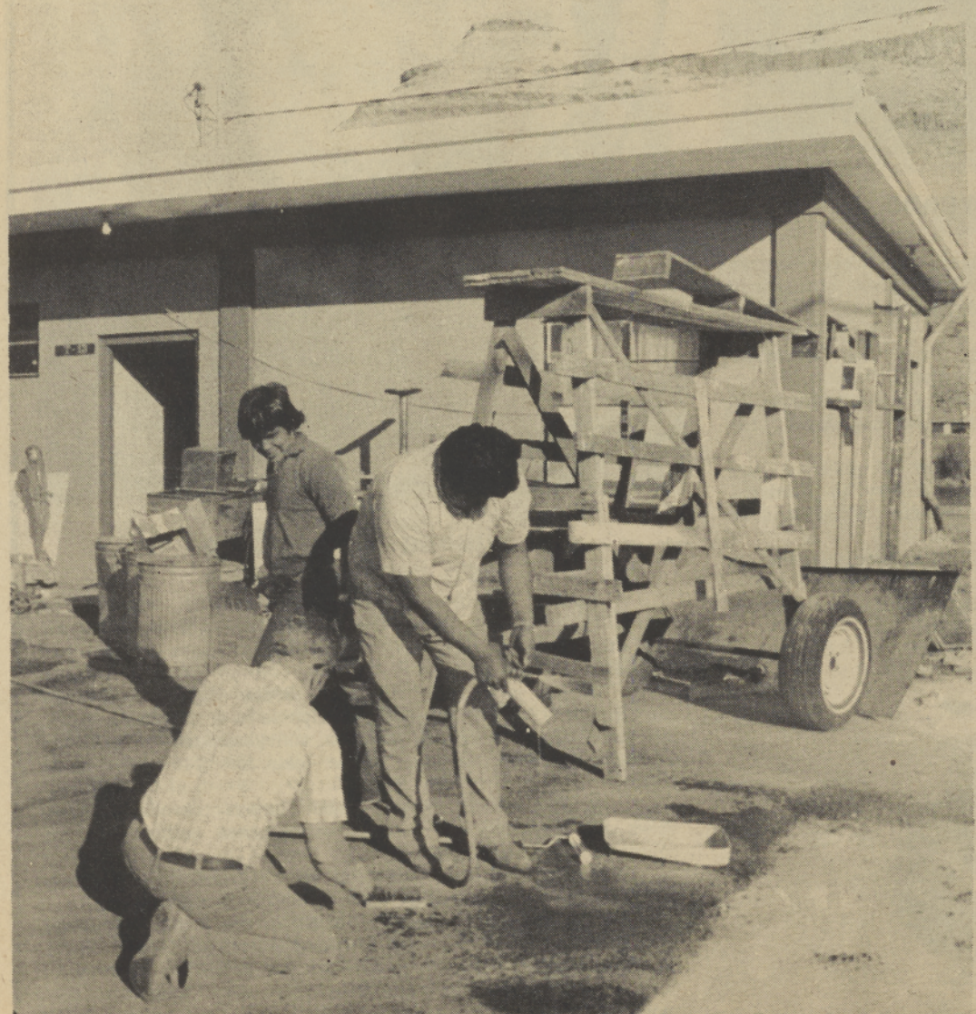
Alice's Restaurant got a facelift last week when Tribal Utilities plastered, painted and repaired the building which is a Tribal rental. Onan Beasley (kneeling), Alvis Smith, Jr., and Lester Tanewasha were found by Spilyay at quitting time cleaning their brushes.
