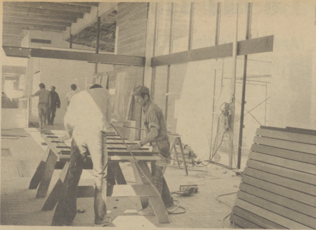
With the new administrative center nearing completion, here unidentified carpenters assemble sections to be used in the new Tribal Council chambers. Photo by Sandy Rangila
