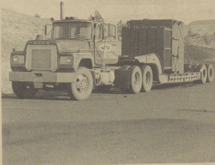
THE NEW TRANSFORMER, which was trucked from Umatilla after the old one blew up, sits in front of the lodge waiting for the crane.
