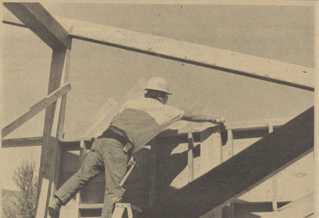
LARRY ARTHUR, shown taking a roofline measurement, is one of the several local men working on the Warm Springs Information
