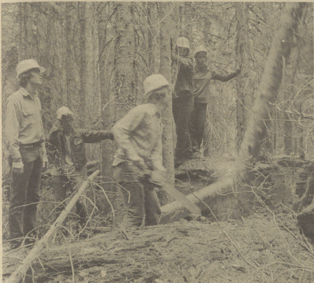
ONE OF THE Y.C.C. crews falling a tree for material to build a bridge across the creek on
