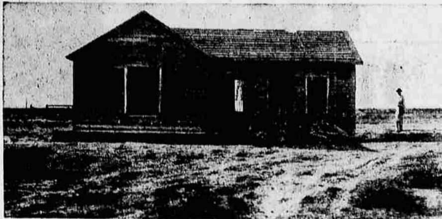
This house, abandoned and falling to pieces, stands on the eastern Colorado plains subject to the ravages of sun and wind, drought and dust.
