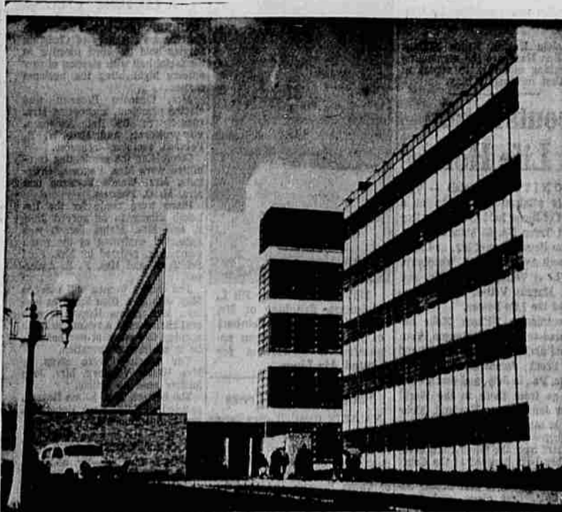
Hundreds of aged persons are housed in this modern geriatrics building—the newest of the institution. The maximum amount of light is available in the interior because of the large percentage of glass in the exterior walls.
