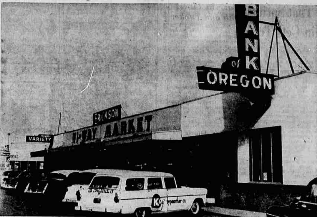
Recent expansion of Woodburn has seen this development along highway 99E. Located here in modern structures are a locally owned bank, food markets, automobile agencies, motels, stores and factories. This is the part
