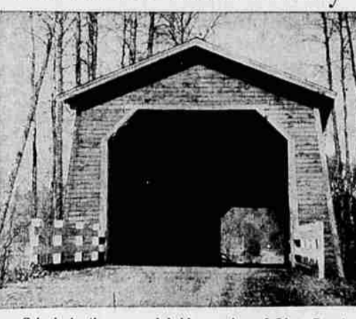
Scio is in the covered bridge region of Linn County. Here is pictured the Shimanek bridge which was named for a Czech family which lived in the community some time ago. The bridge is 35 years old.
