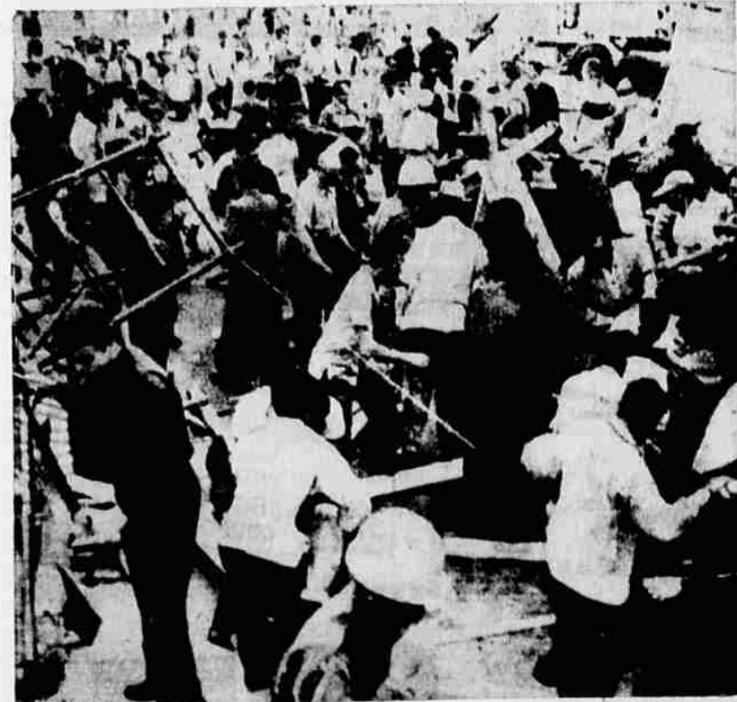
HAVANA, Cuba—Spectators and police rush in to lift wreckage aside and drag the injured to safety yesterday after wood pedestrian bridge collapsed. Ten persons were reported seriously injured in more than a score of people crowded it to watch start of Grand Prix race qualifying trials. Bridge was temporary structure over the Malecon, boulevard in Havana used as route for sports car races. (AP Wirephoto).
