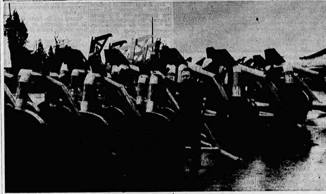
The two pictures above show the town of Independence and the proprietor of its largest industry. The top photo shows Main street. Down the street can be seen the home-owned and home-operated First National bank, started by Joe Hirschberg in 1889. The lower picture shows Mayor Francis Holt with some of his agricultural and logging equipment. Holt is proprietor of Independence's largest industry, which provides work for 110 employees. (Capital Journal Photo).
