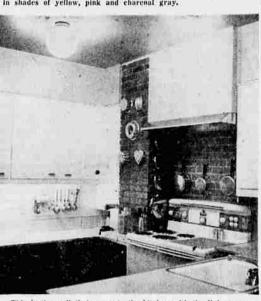
This is the wall that connects the kitchen with the living room. It used to be cupboards, but Don Dill investigated, found a brick chimney so tore down the other wall and, by slicing bricks, com-pleted the rest of the wall in brick. He put over the stove a copper funnel to draw up cooking odors.
