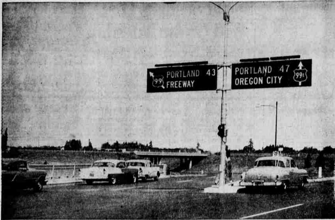
AUGUST 10 — Opening of the completed Baldock Freeway to Portland was major highway news locally of 1956. The four-lane route cuts driving time to Portland by several minutes. Freeway opening headed news of giant Federal-state highway construction program which will provide new roadways throughout the state.
