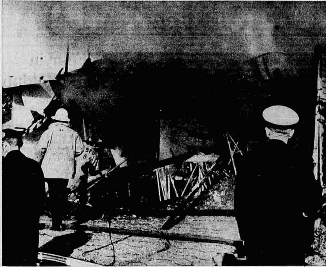
Firemen and spectators view remains of the Dennis Howarth home 785 North 20th St., which was destroyed by an explosion Wednesday morning. Mr. and Mrs. Howarth and their daughter, Decann, 5, were reported in "fair" condition at Salem General hospital. All three were blown out of the house by the explosion. They suffered first, second and third degree burns.
