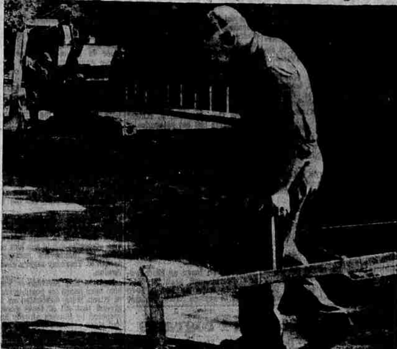
One of the first jobs necessary when work began on tearing down the old wooden bridge on South High street early this morning was locating all underground pipes and utility lines with an electronic device here handled by John Keller, foreman of the crew. Other preliminary work to replacing the old structure with a modern concrete bridge was tearing up the old boardwalks along each side. It will take nearly a year to finish the job.
