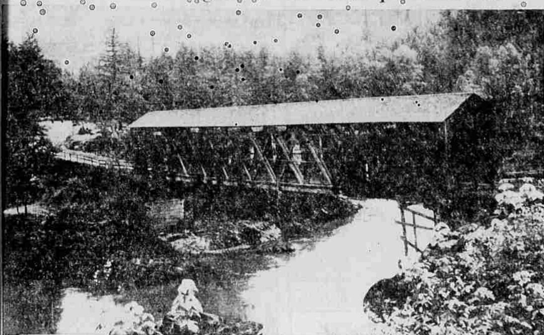
When the old covered bridge spanning the North Santiam gorge between Marion and Linn counties at Gates was razed in 1938 residents of the community regretted the passing of a structure regarded as one of the more picturesque of its kind in Western Oregon. Gates covered bridge was built in 1902 and had a span of 174 feet.
