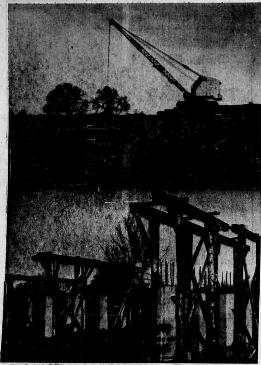
Top: Concrete bridge now under construction by the C. J. Aldon Co. of Portland will carry the new North Santiam highway across the Mill creek diversion channel recently opened immediately east of Salem. This structure will be 200 feet in length with a 30-foot roadway. Five men are now employed on this job. Lower: Overcrossing of reinforced concrete that will carry the North Santiam highway over the East Salem by-pass route a half mile south of East State street. This overcrossing will be 190 feet in length.
