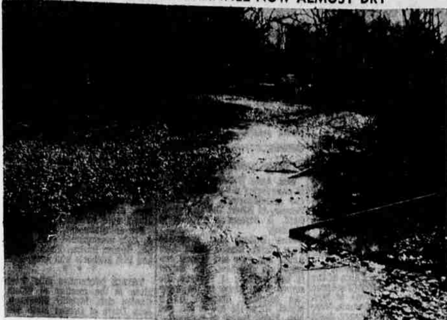
A recently constructed diversion channel for Mill creek near 5550 feet in length has practically drained an old, established channel of the stream in an area that was a favorite Salem picnic locality 25 years ago. At the point shown in this picture New East Salem bypass route will bridge the stream's bed. A token flow will continue through the old channel during most months of the year.
