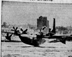
The R3Y, Tradewind, America's first seaplane transport powered by jet engines turning propellors, alights on San Diego bay after its initial flight. Arrow points to the No. 2 engine which was feathered because of the malfunction of a small governor in the powerplant system. Consolidated Vultee Aircraft Corp. is building the plane for the Navy. (AP Wirephoto)
