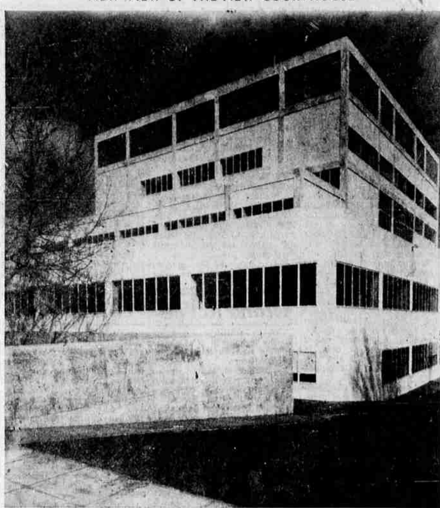
This photograph of Marion county courthouse, now nearing completion, was made with aid of a strong filter to show marble texture and differentiate planes of the structure as they appear from the south driveway entrance on State street.
