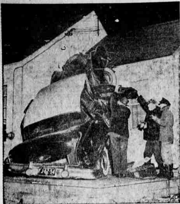
Grand Rapids, Mich., deputy sheriffs examine wreckage of an automobile that leaped up the concrete porch and smashed into the side of the John Dewey residence, shoving the house six inches off the foundations. Car hit the side of the living room just vacated by the Dewey family. The driver of the car is in fair condition. (AP Wirephoto)
