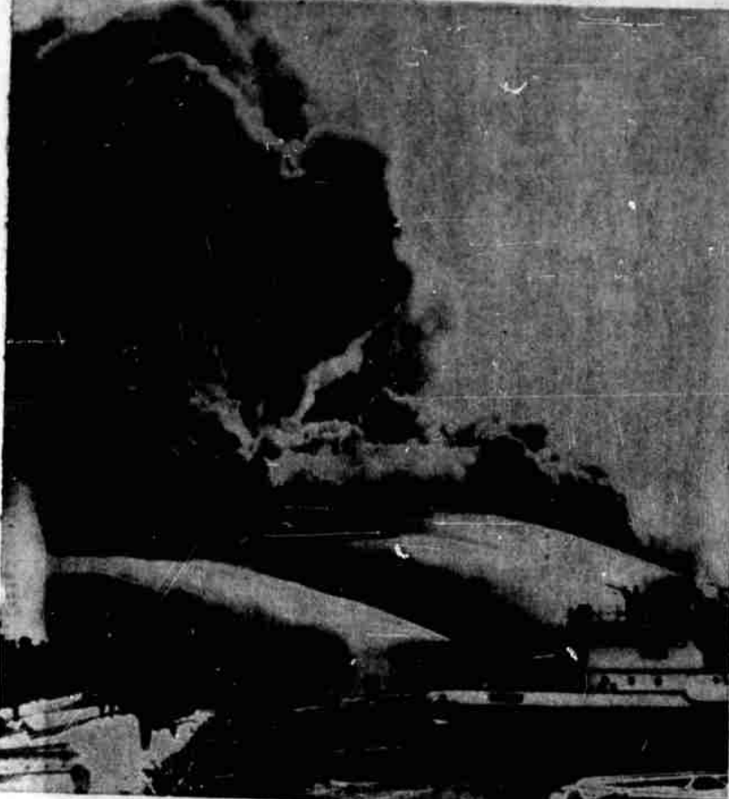
New York, Jan. 15—Dense smoke rises from four historic warehouses along the Brooklyn waterfront here today as spectators, left, watch firemen pour streams of water into the structures from a fireboat. The warehouses once were used as ammunition depots in the Civil War. Twenty-one firemen were injured, most of them by falling debris when a wall gave way. Damage was estimated at $3,000,000. (AP Wirephoto)
