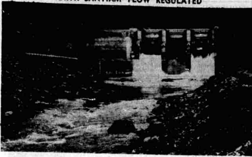
Two spillways on the Big Cliff dam on North Santiam river are now in operation. The dam is situated down stream from Detroit dam and is used to regulate the flow of water released from Detroit lake. Concrete structure at left of dam is power house not yet equipped for operation.
