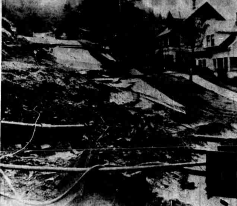
Astoria, Ore., Jan. 7—Fifteen families abandoned their homes and eight others prepared to do so as a hillside began sliding here after heavy rains. The slide buckled streets and exposed and broke water pipes shown here. (AP Wirephoto)
