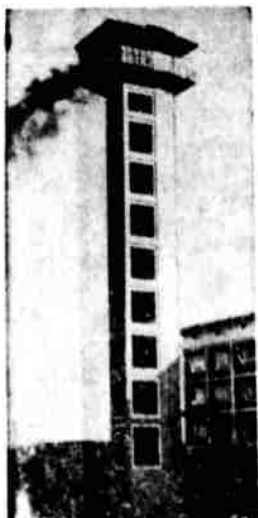
IN DISGUISE — Observation tower in Offenburg, Germany, is in reality a printer's plant chimney which was masked and decorated to make it attractive to sightseers.
