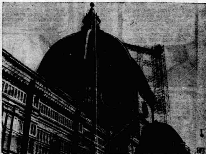
THE DUOMO GETS SHAMPOOED — The Duomo, Santa Maria del Fiore, world famous Florentine church designed by Arnolfo di Cambio in the 13th century, is covered with scaffolding as workmen give its tiled roof a general overhauling to remove ravages of time.
