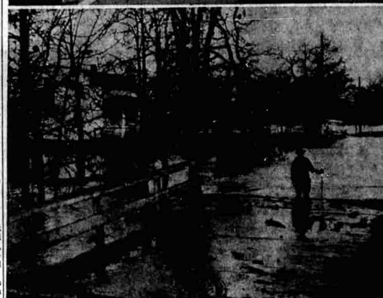
Top photo shows backwaters of Santiam river south of the Jefferson bridge crossing highway and approaching new dwelling at left. Lower photo shows J. C. Bentley standing hip deep in water by washed-out bridge, as flood isolated his house, seen through trees, and barn.
