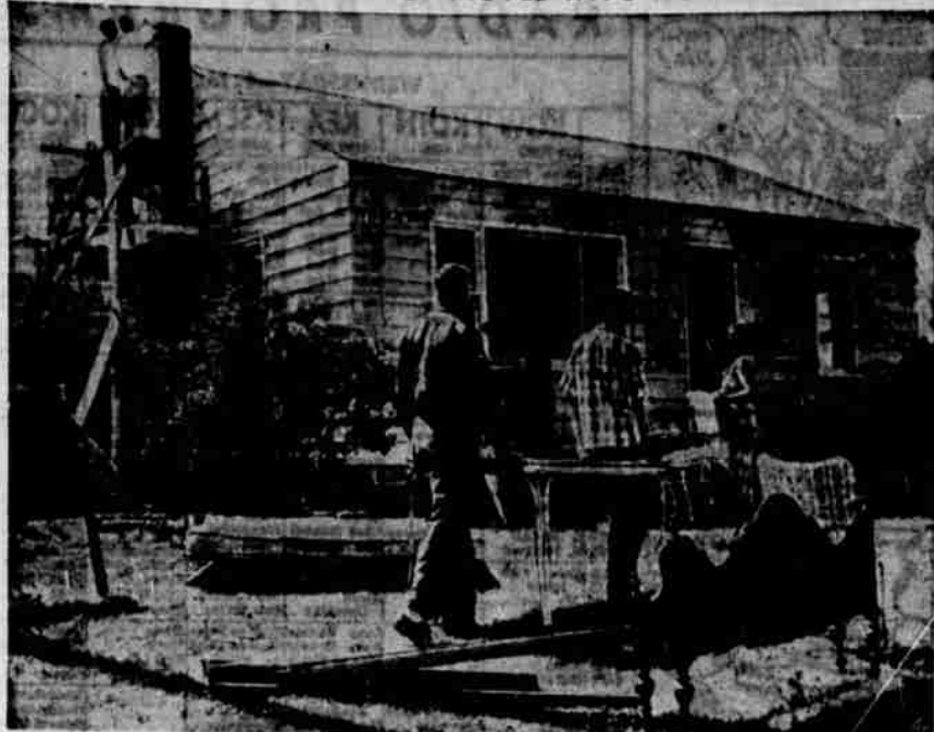
The Allen R. Crosley family moves furniture into their new home at Flint, Mich., while workmen still were putting the finishing touches on. The workers are part of several thousand who pitched in to rebuild 186 homes destroyed by tornado, in "Operation Tornado." (AP Wirephoto)
