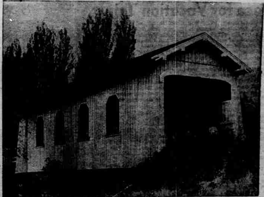
Mill Creek covered bridge on the Alsea highway immediately east of the guard station is the last covered bridge in use on a primary state highway. It has been ordered removed after 29 years of service and will be replaced by a concrete viaduct. Event of the automobile and use of weather resistant concrete in bridge construction has ended the era of these horse and buggy relics in Oregon.
