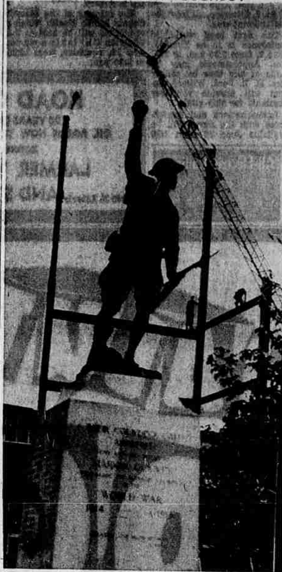
Erection of upper floor steel for new Marion county courthouse created this frame for the county memorial to veterans of first world war. Practically all structural steel needed for courthouse construction is now at hand.
