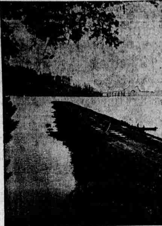
The old Hauser-Coos Bay road in southwestern Oregon climbs around the head of Haynes Slough between Hauser and the bridge for 6.38 miles. The new highway wades right across the mouth of Haynes Slough to hook onto the end of the Coos Bay bridge, is 4.55 miles long, saves 1.83 miles and has but nine curves compared with 60 on the old route. It is a time and money saver. (State Highway Commission photo)
